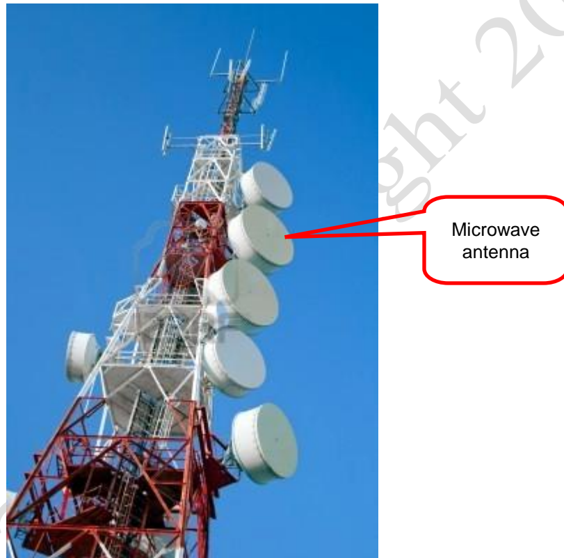
Figure 10.7 Microwave antennas with reflectors on a tower
